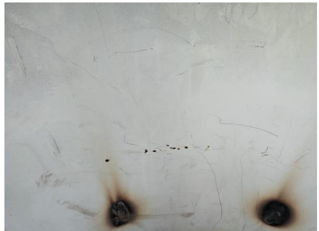
Pinholes through dry riser tube
